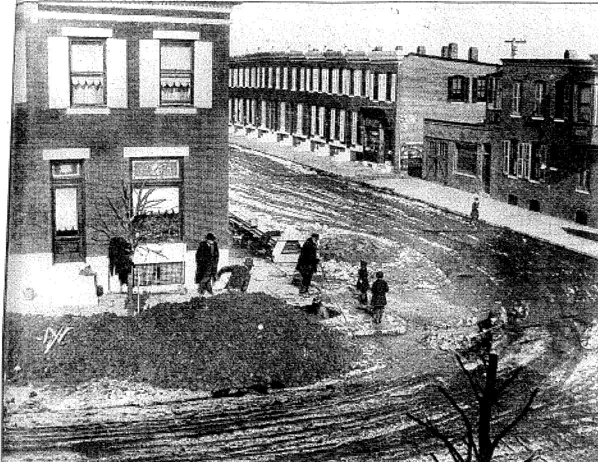
Sewer hookups were done largely with manual labor, which continued despite harsh winter weather. This shot from the 1920s was taken at Hudson and Dean Streets. (Courtesy John Rockstroh.)
